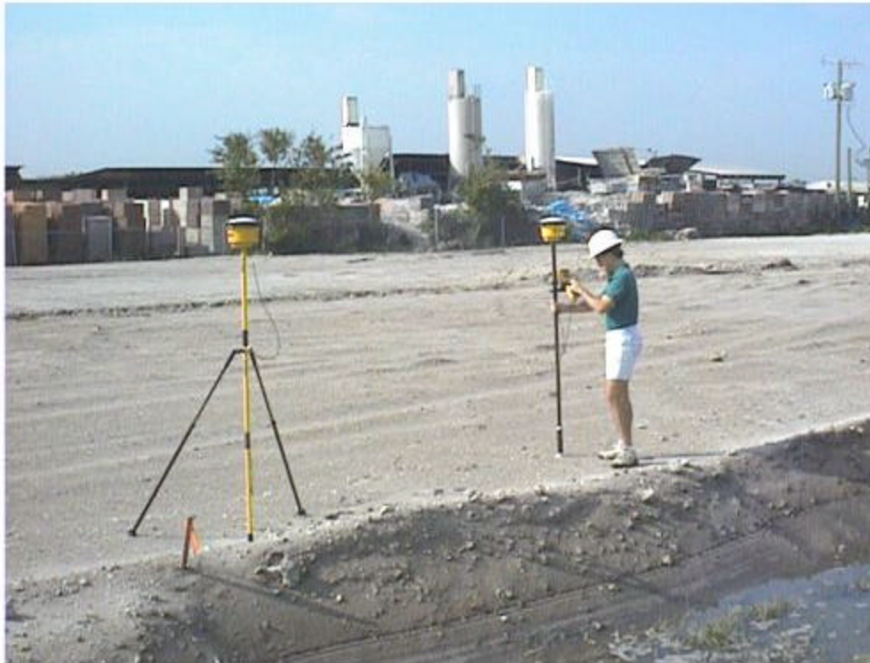
Figure 9-15. Real-Time kinematic survey reference and remote stations
