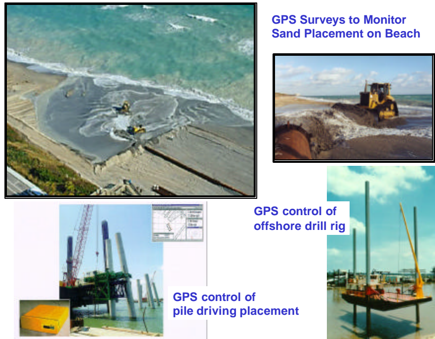
Figure 6-11. Construction grading and core drill location GPS applications
